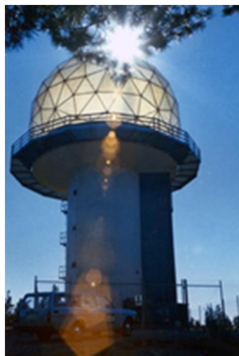
Radarstation PS-810 (Foto FHT)
